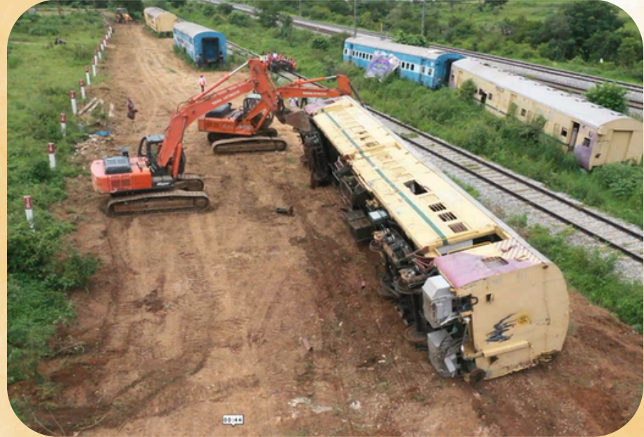
UTILIZING ROAD-MACHINERY IN RESTORATION
