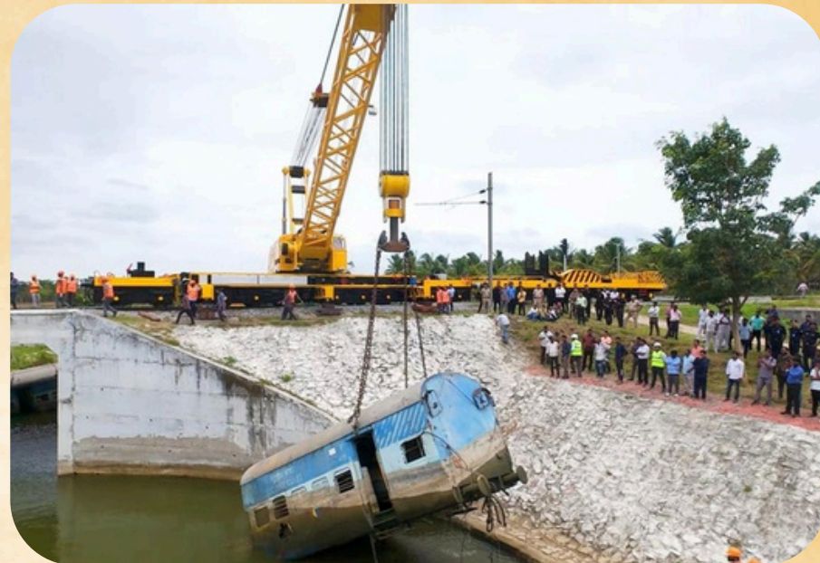
RAIL CRANE BASED RESTORATION EXERCISE
