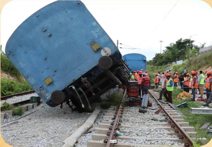
COACH TOPPLING WITH HYDRAULIC RERAILING EQUIPMENT
